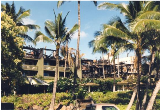
THE BUILDING AFTER THE FIRE
